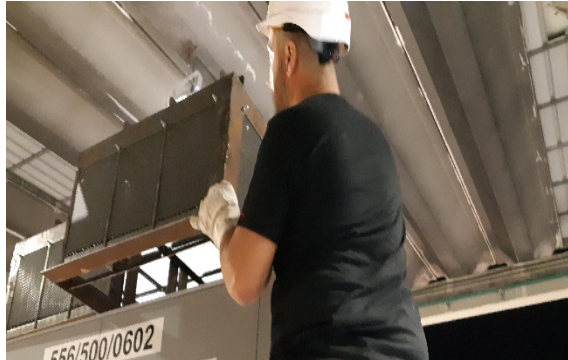
Fig. 10. Mounting of box-shaped honeycomb ventilation panels on the DG casing's roof.
