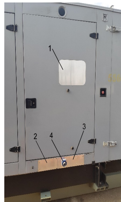
Fig. 2. Metal plates mounted into cut-offs in the medium-capacity DG casing. 1 – in front of main controller's window; 2 – detachable panel for power cables; 3 – permanent panel with a power connector 4 - to connect 220V power cable running between the internal charger and the external 220V line.
