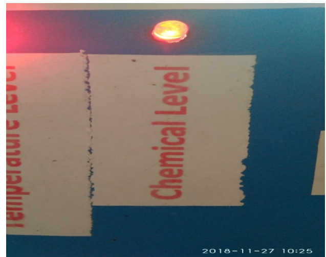
Figure-5: Chemical tank
