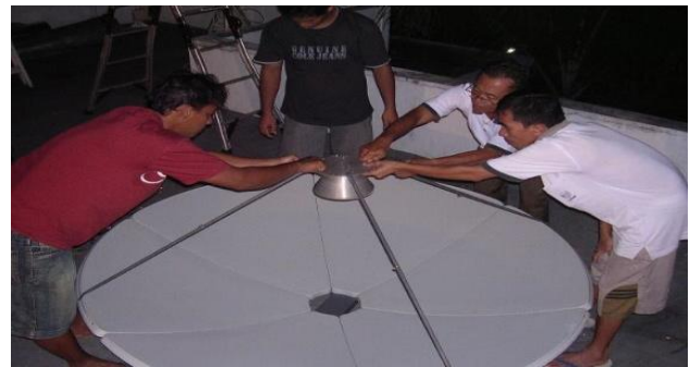
Figure 9. Install Feed Horn on Parabola
