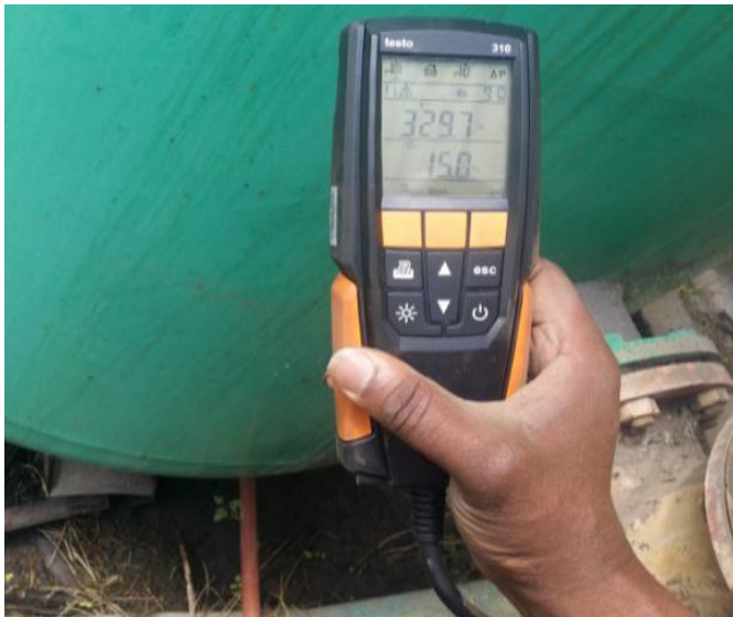
Figure 5: Flue gas analyzer data measurement for wood fire-tube boiler
