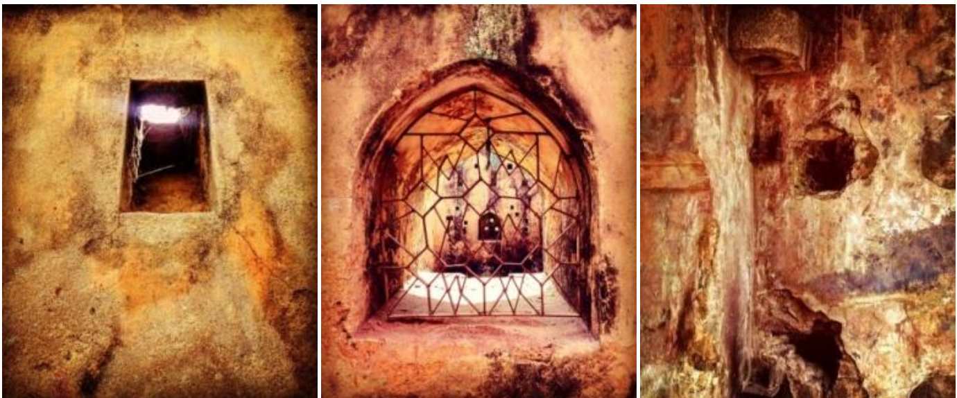
Figure 30,31,32 Shows:: Detailed description of the defensive wall of Sonakanda Fort.
