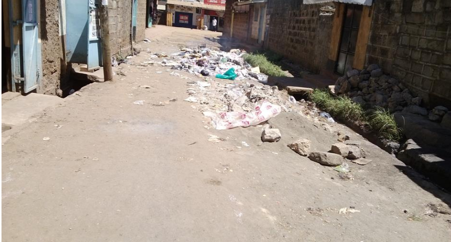
Figure 5.8.2 : Open dumping of wastes on an access road in the town.
