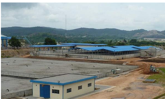
Figure 1. Lower Usman water treatment plant in Bwari Area of FCT, Abuja.
