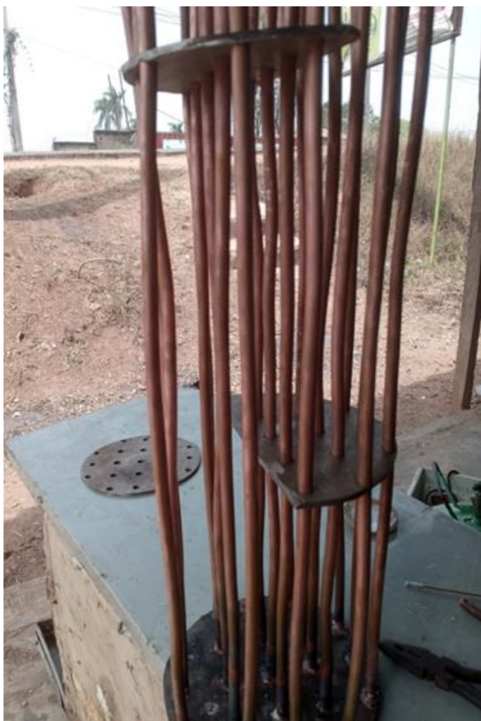
Plate 2: Construction process of the tubes on the tube plate and baffle
