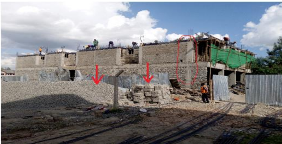
Figure 6: Material delivery to construction area
