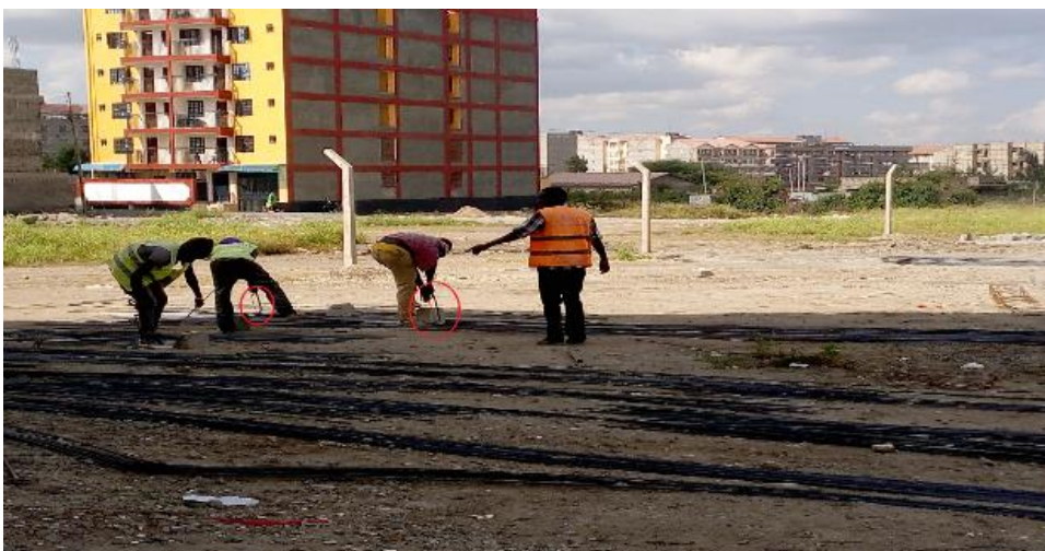
Figure 7: Cutting reinforcement steel using hand tools.
