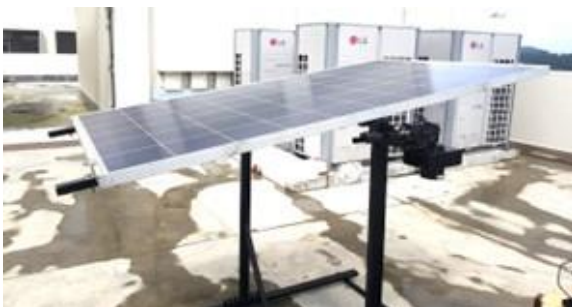
Fig 2: Developed solar PV mounting structure
