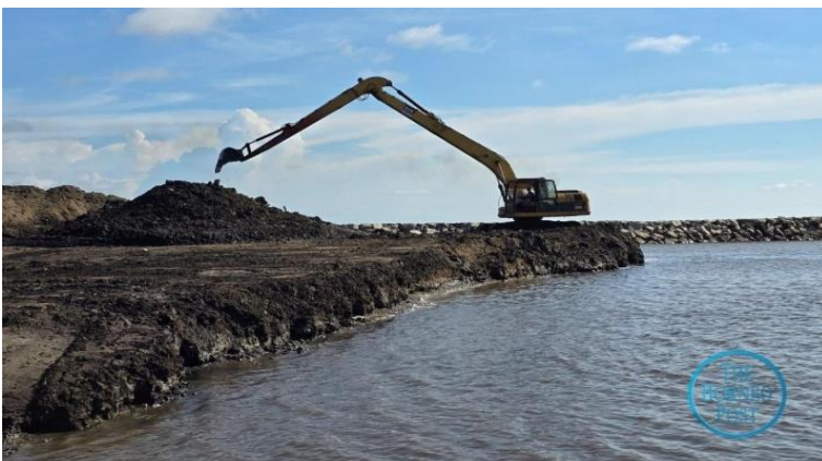
Figure 2: Ongoing excavation work at Kampung Batu Satu to remove sediment buildup by the coastline.
