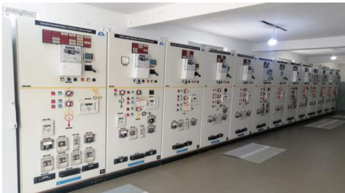
Fig. 2 Atoabo Substation 33 kV Indoor Panels
