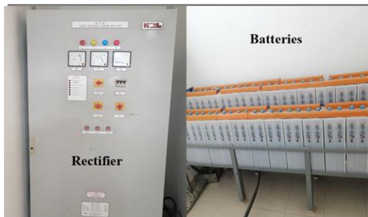
Fig. 4 Atoabo Substation Rectifier and Batteries
