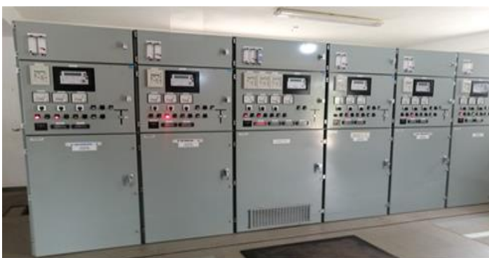
Fig. 3 Atoabo Substation 11 kV Indoor Panels
