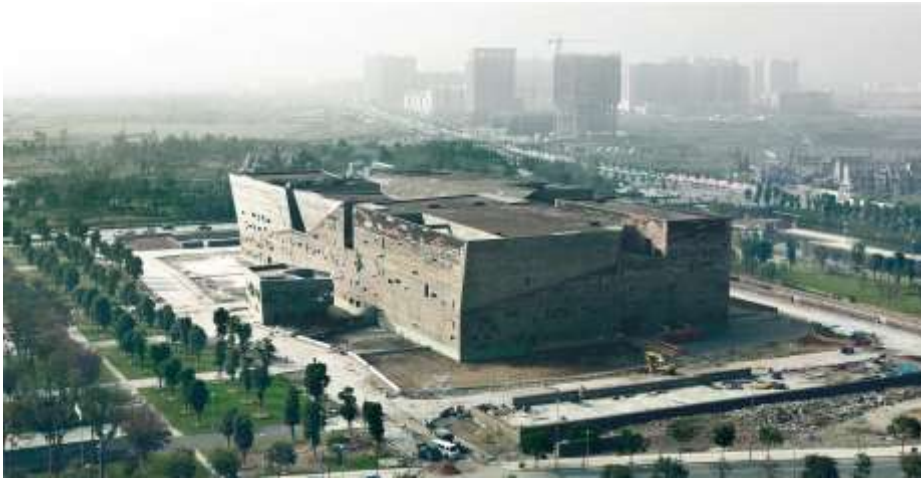
Figure 27. The Ningbo Museum, Yinzhou District, Ningbo, China, 2008 (Architect: Wang Shu)
