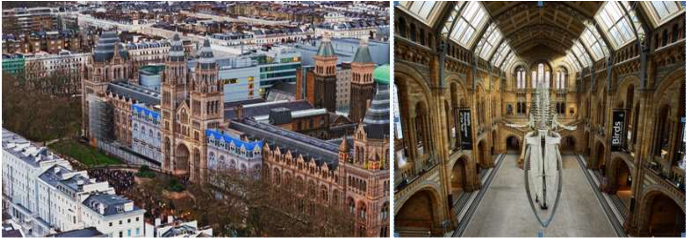
Figure 22. Natural History Museum, London, United Kingdom, 1881 (Architect: Alfred Waterhouse)
