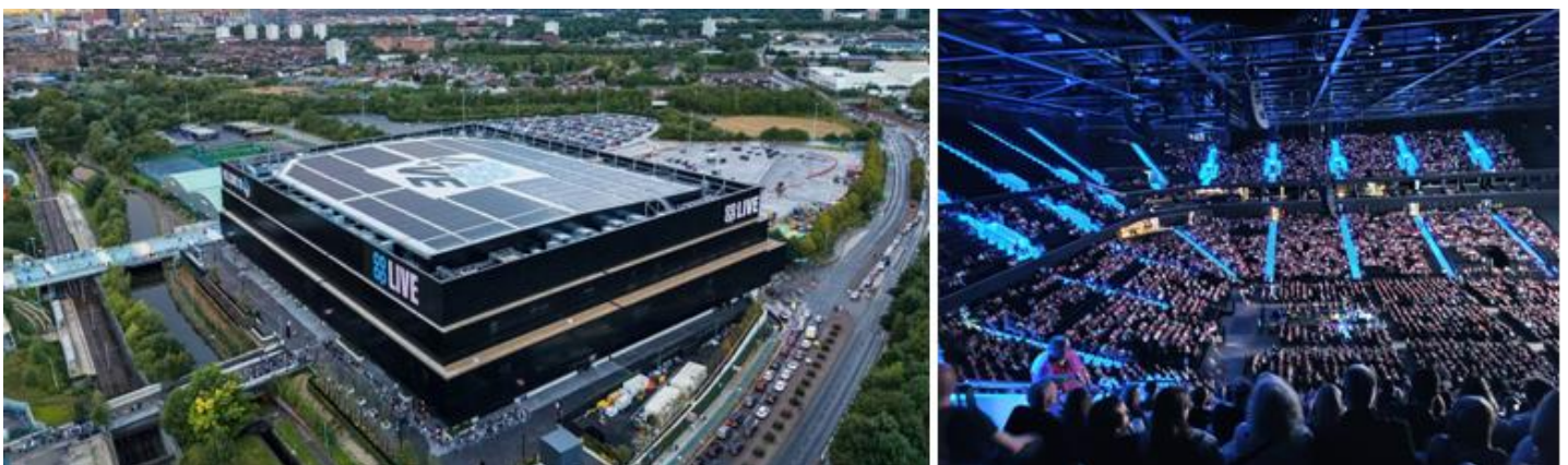
Figure 4. Co-op Live, Manchester, United Kingdom, 2024 (Architects: Populous)
