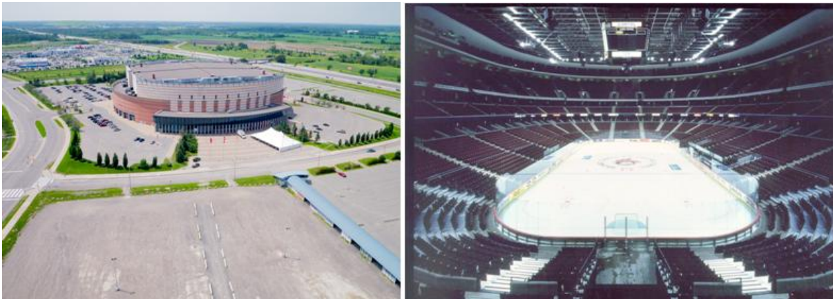
Figure 18. Canadian Tire Centre, Ottawa, Canada, 1996 (Architects: Rossetti Architects Murray & Murray Architects; Structural engineer: Carruthers & Wallace Ltd.)
