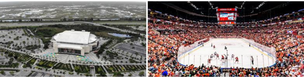
Figure 15. Amerant Bank Arena, Sunrise, Florida, United States, 1998 (Architect: Ellerbe Becket; Structural engineer: Walter P. Moore & Associates)
