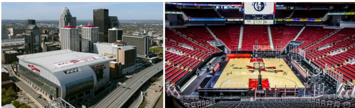
Figure 10. KFC Yum! Center, Louisville, Kentucky, United States, 2010 (Architects: Populous (formerly HOK Sport), Louis and Henry Group, C.L. Anderson Architecture, Jill Lewis Smith Architects)
