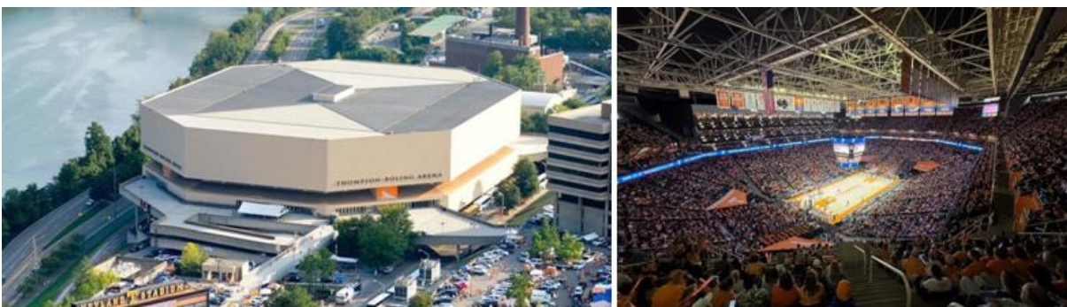
Figure 13. Thompson-Boling Arena, Knoxville, Tennessee, United States, 1987-2007 (Architects: GSCD, Inc. Architects, Cideco Architecture & Planning Inc.; Structural engineer: Ross H. Bryan Engineers Inc.)
