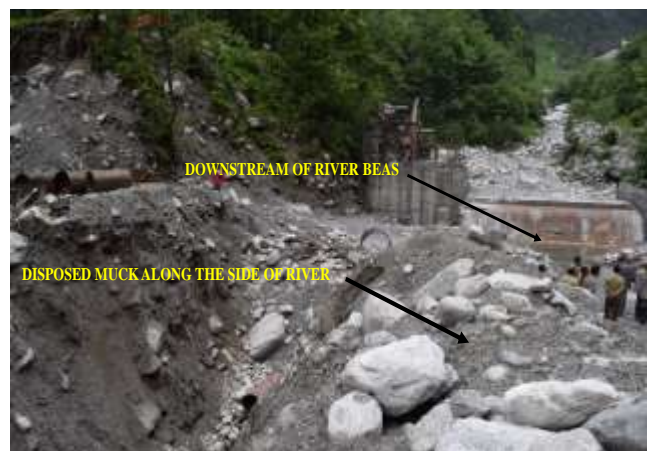
Figure 3: Muck disposal along the side of River Beas.
