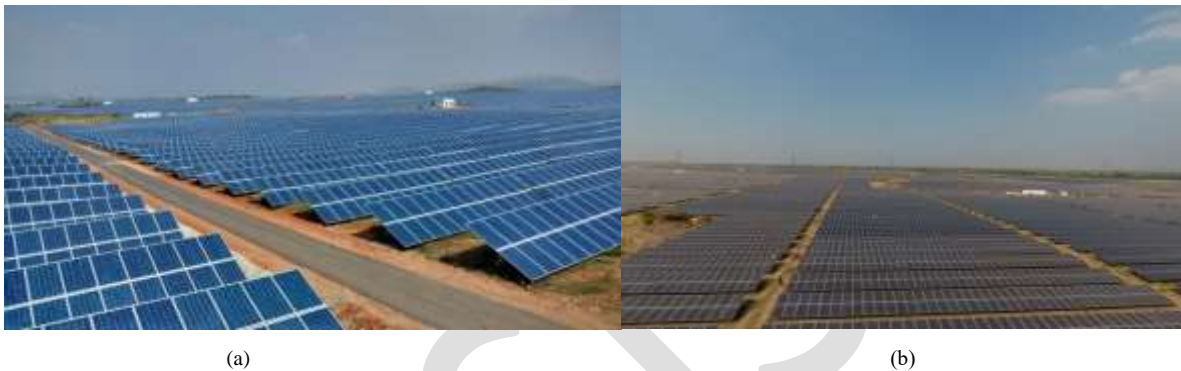
Figure 2 (a) Ananthapuramu Solar Park (b) Kurnool Solar Park
