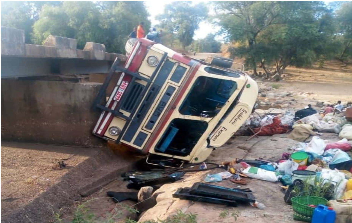
Picture D- Bus fell off the narrow bridge
