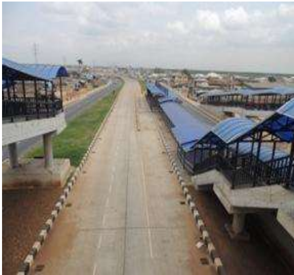
Plate2: Bus Rapid Transit (BRT) Line/Terminal in Lagos/Ikorodu Road
