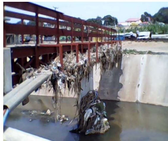
Fig.7 Trapped rubbish on a foot bridge across the Odaw River from Tesano to Alajo indicative of the amount of waste carried by the river when in spate
