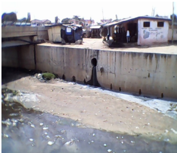
Fig.4b Siltation of the Odaw River at the bridge from Tesano to Aladjo
