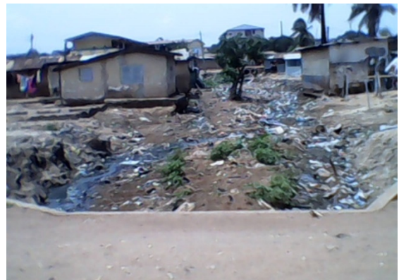
Fig.5b Unconstructed drain filled with rubbish
