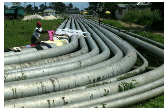
Fig 1: A typical stretch of Oil Pipeline
