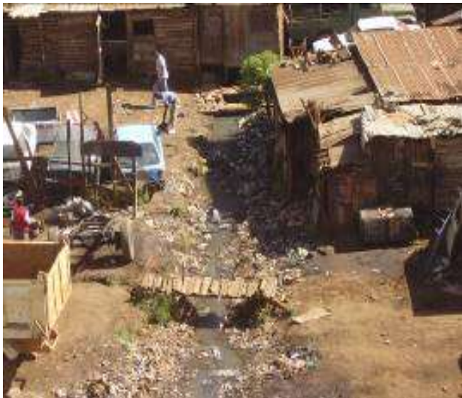
Figure 1. Waste Disposed in Drainage System
