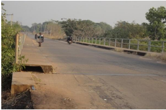
Figure 6. The completed River Konshisha bridge leading to Tse-Agberagba (January, 2017).
