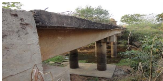
Figure 5. Under view of uncompleted Selagi bridge across River Konshisha (January, 2017).
