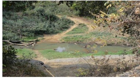
Figure 4. Propose Bridge Point at Dio-Mbatwer (January, 2017).
