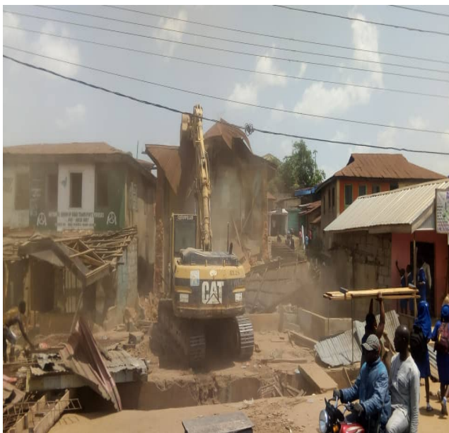
Figure 3: The demolition of affected residential building for the Flying Over
