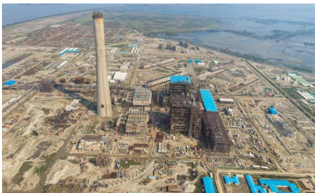
Fig. 8. Present scenario of the Rampal power plant project
