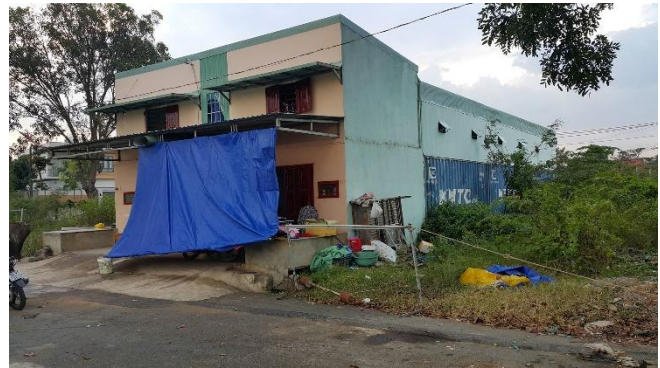
Fig. 8. A house made from bricks, metals, and old containers for adjacent rooms for rent in District 9, Ho Chi Minh City (SUD 2017, 2017)
