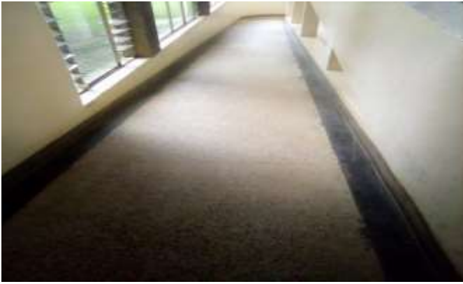
Plate 1.1 Accessible Classroom with ramps
