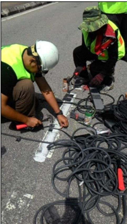
Figure 12: Spiked down of each tube (through the C-clamps)
