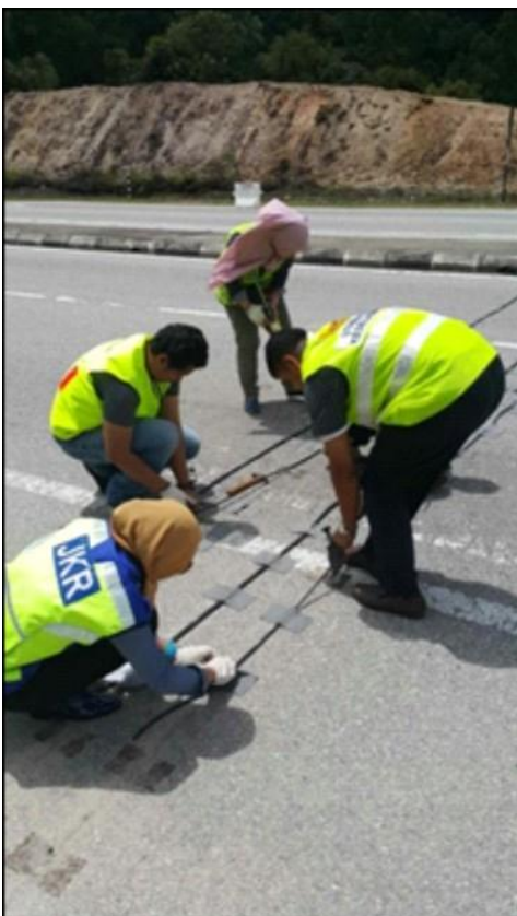
Figure 16: During the uninstallation of road tube
