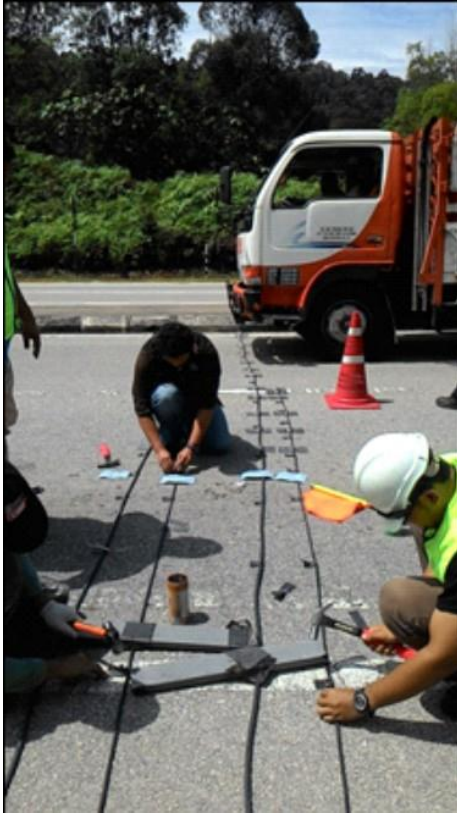
Figure 8: The traffic flow between lane are separated by cone
