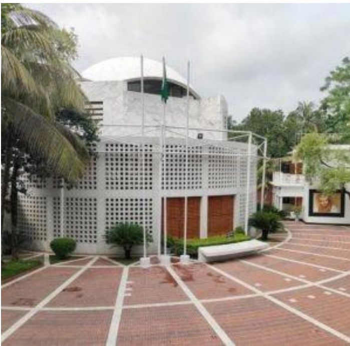
Figure-3: Study location of the selected area (Bangabandhu’s Mausoleum, Tungipara, Gopalganj)
