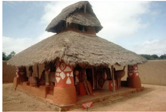
Plate 1: A shrine finished with mud plaster, thatch roof, and decorated with natural dye (uli paintings) in Imo State.
