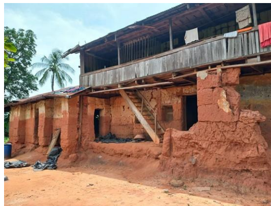
Plate 2: one-story building finished with mud and timber in Aniwa-olu, Delta State
