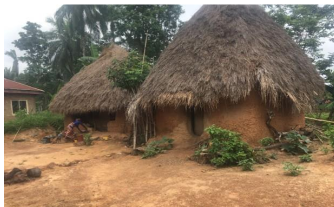
Plate 3: A hut in Ebonyi state plastered with Mud and thatch
