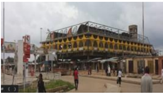
Fig. 5a: Jos Ultra-modern market before bombed
