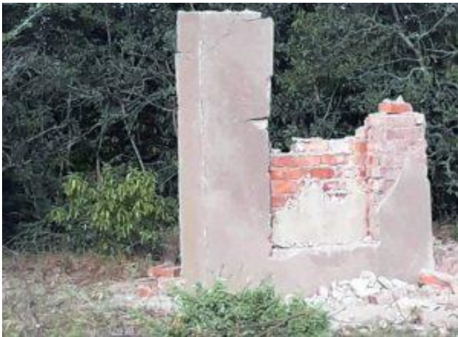
State-destroyed Bhalagwe plague.
