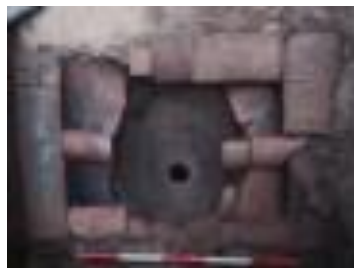
Figure 56 Bathing room drain.
