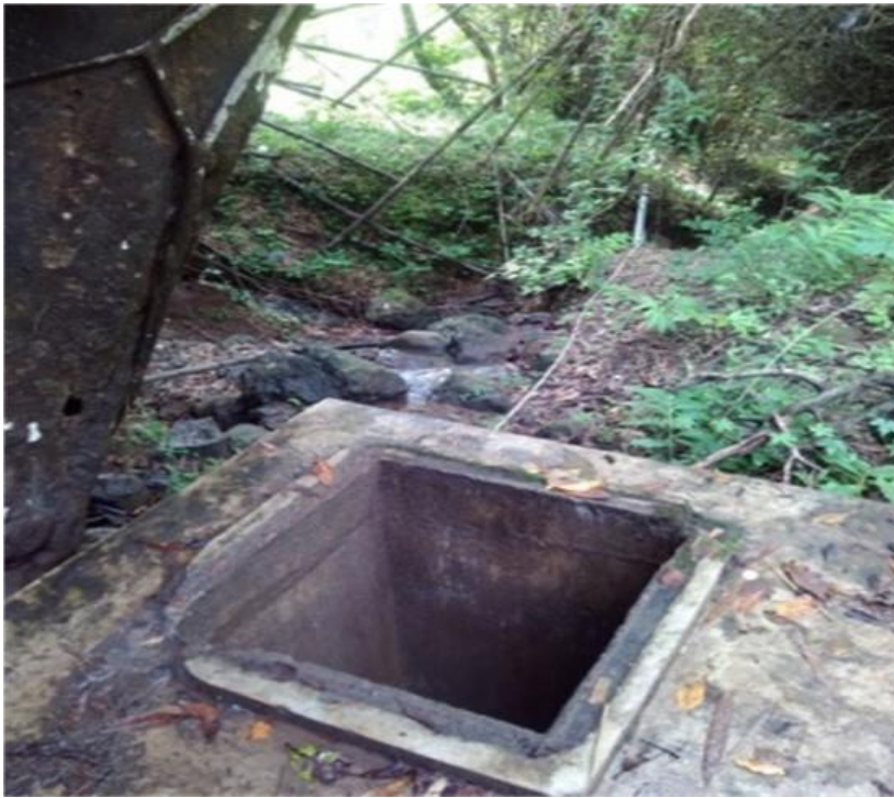
Figure 2: Mount Budheg Spring Water Storage Tank in 2011, Source: LMDH Wono Yoso.
