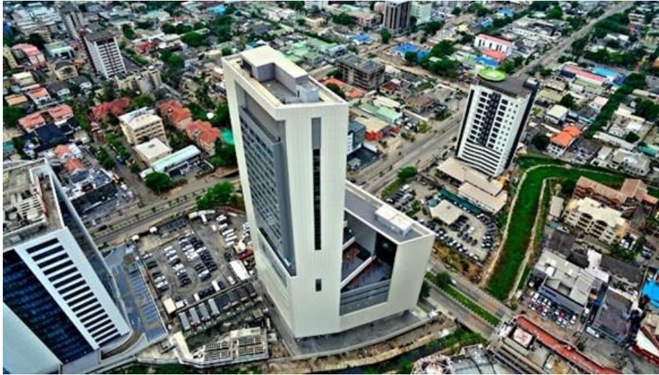
Fig.2:3 showing overview of Eko Tower Complex
