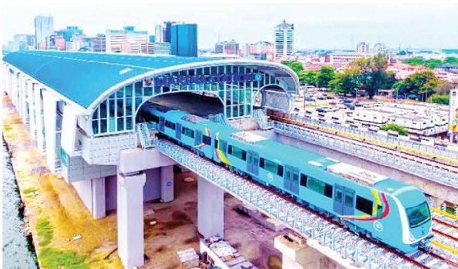
Fig.2: 4 showing the Lagos Light Rail Station
