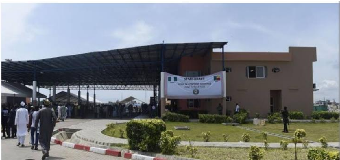
Side View of the Administrative Block
