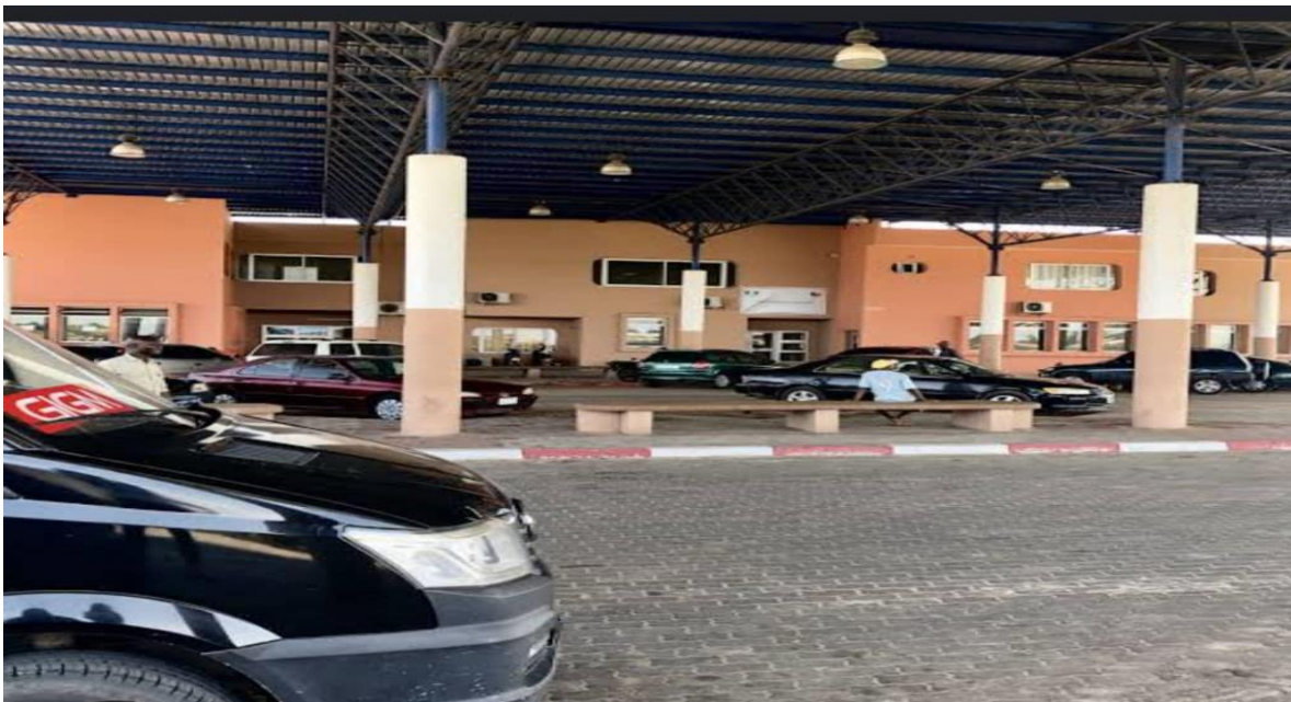
Figure 5 Administrative Block, Seme Border (front view)
