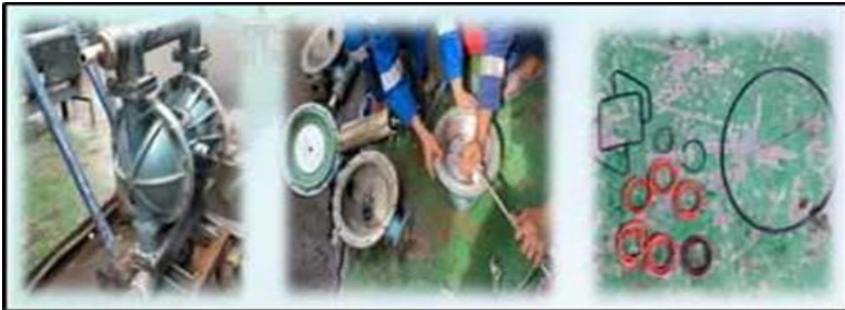
Figure 9. Diaphragm Pump Repair Process
