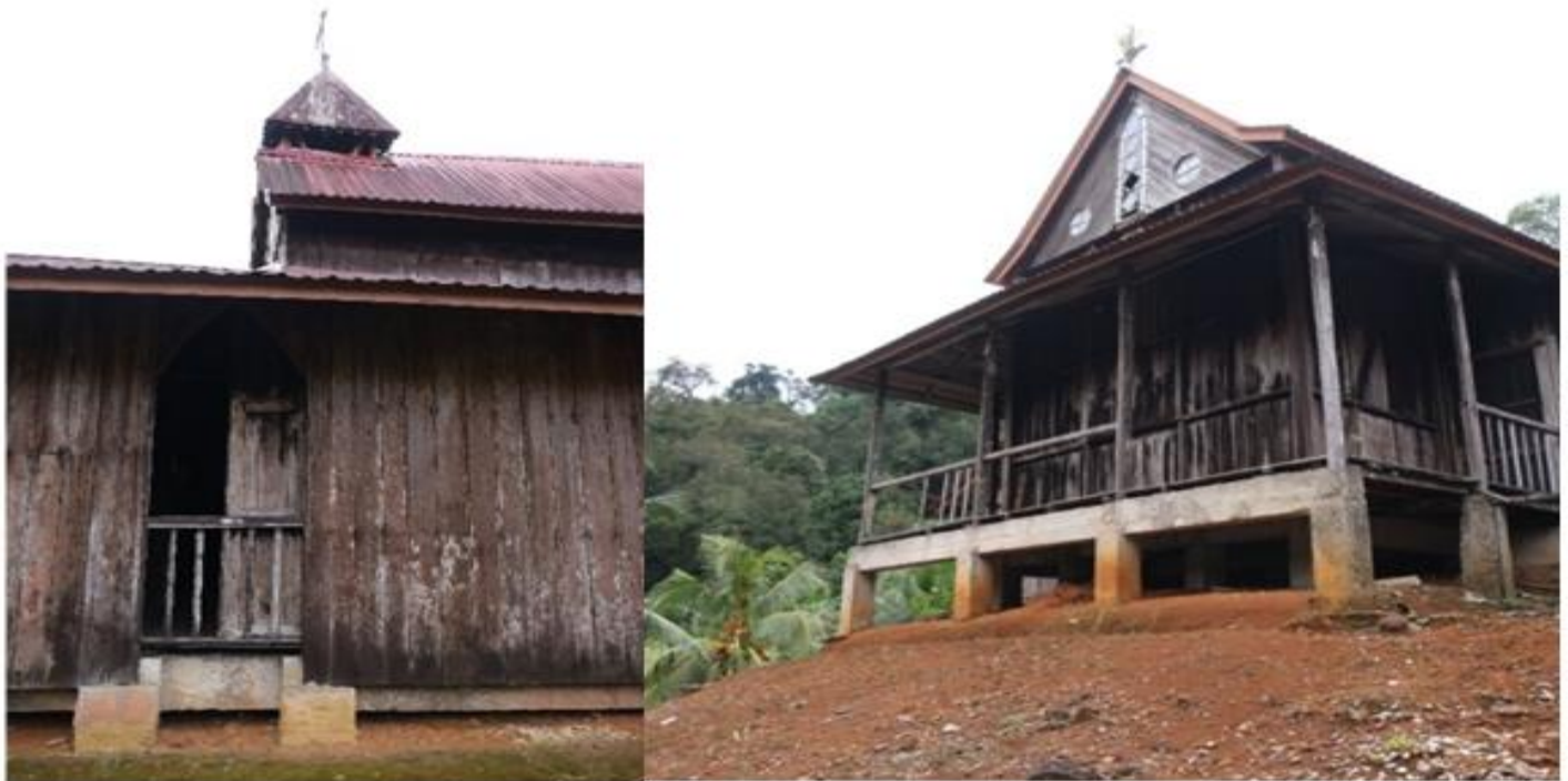
Fig. 6: Raised Reinforced Concrete Strip Foundation of St. James Church, Kampung Quop
