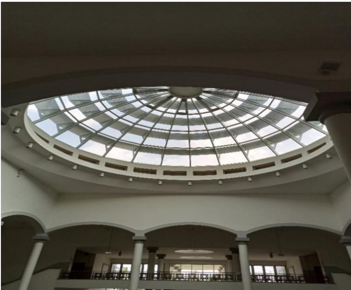
Plate 6: Dome skylight at the atrium of Calabar International Convention Centre
