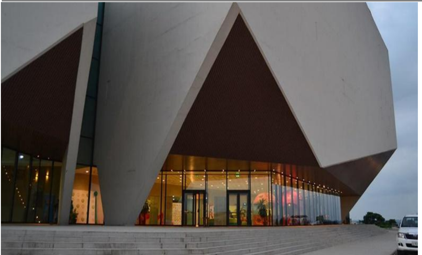
Plate 5: Building envelope and overhang to the curtain wall system of Calabar International Convention Centre
