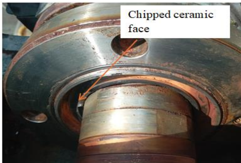
Fig 2. Inspection of the chipped ceramic face
