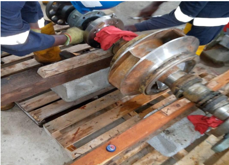
Fig 4. 50-P-007B bearings/ seal removal
