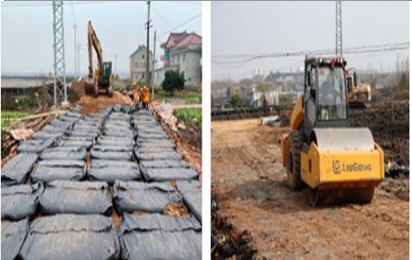
Figure 5: Polypropylene soilbags provide three-dimensional confinement of soils.
