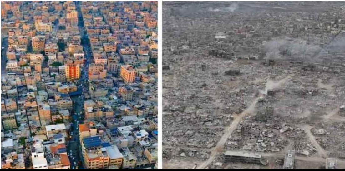
Figure 1: Jabalia Camp in Northern Gaza before and after October, 2023
