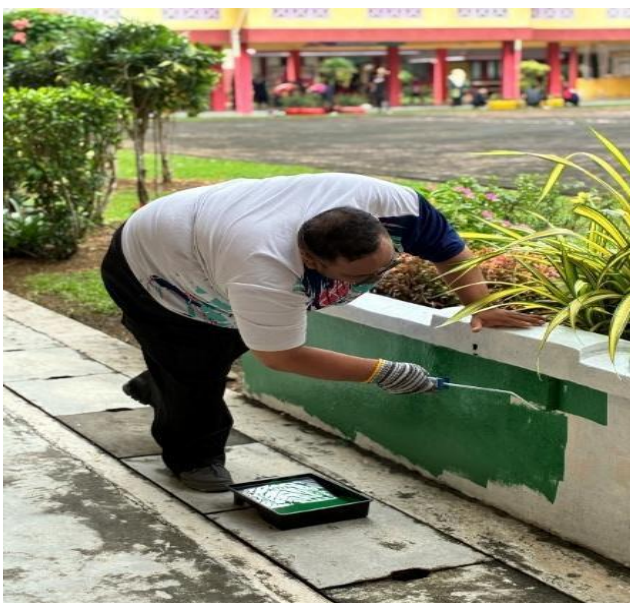
Fig. 6. Wall painting activity around the school environment.
