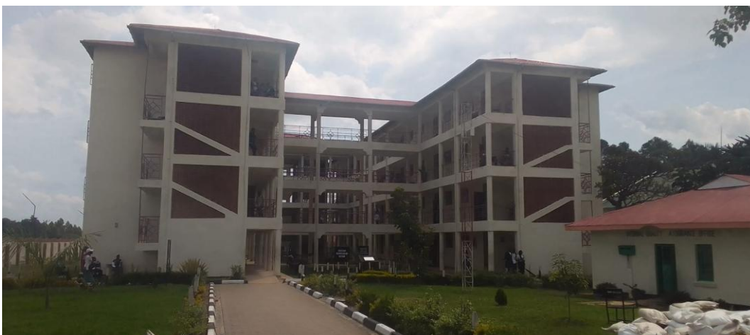
Complete and operational 4 Storey Tuition Block of Institution A FY 2019/2020
