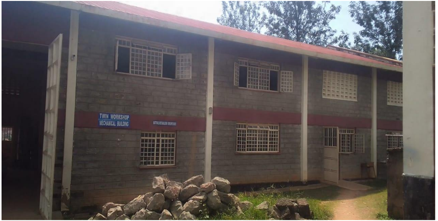
New Workshop Construction of Institution A FY 2020/2021
