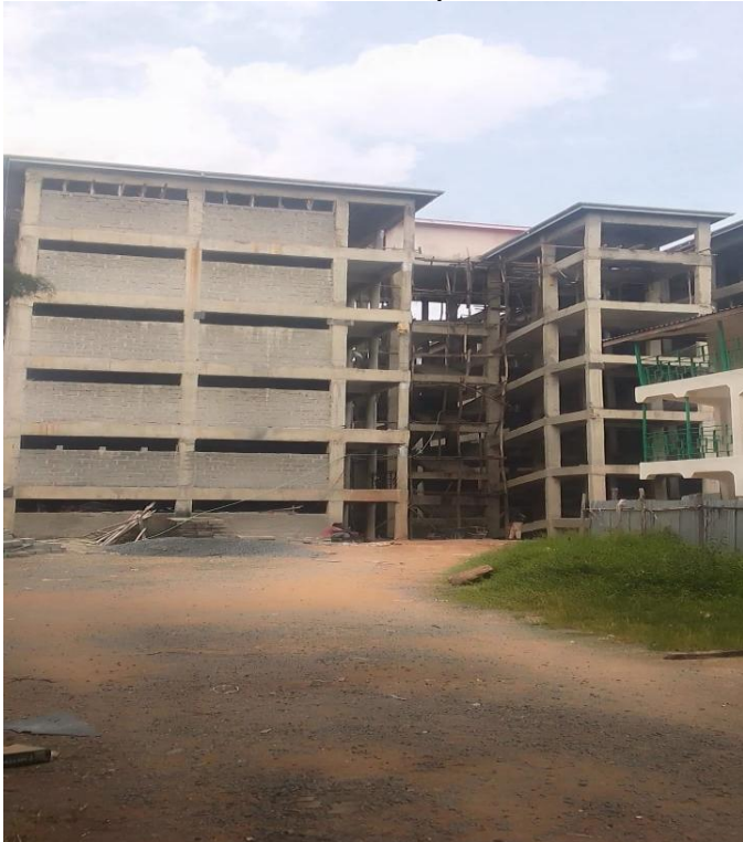
Incomplete 7 Storey tuition block of Institution A FY 2022/2023
