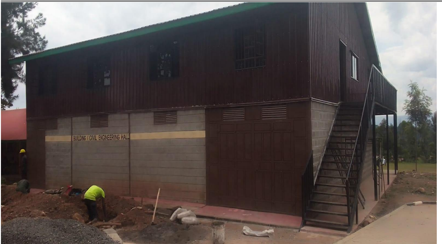
Civil Engineering Hall of Institution D FY 2022/2023
