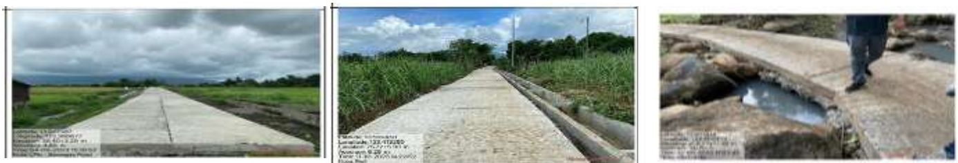
Figure 6. The Completed Subprojects
