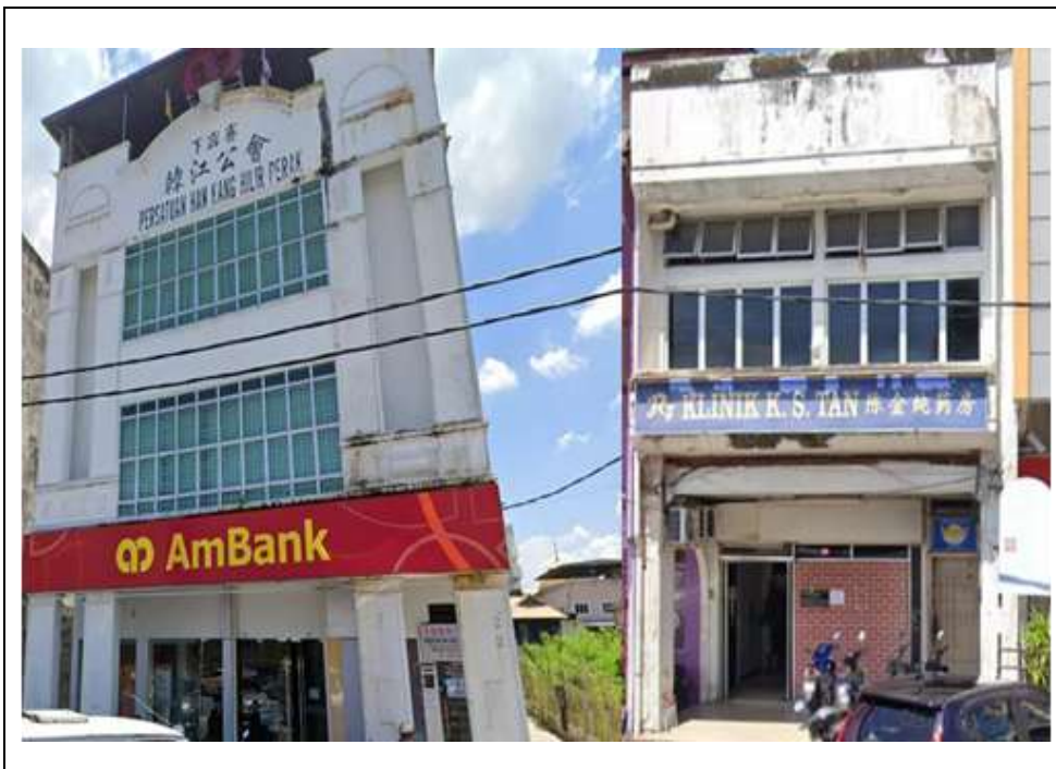
Photo 2: Neo-Classical Style Building Facades (1880s – 1920s)
