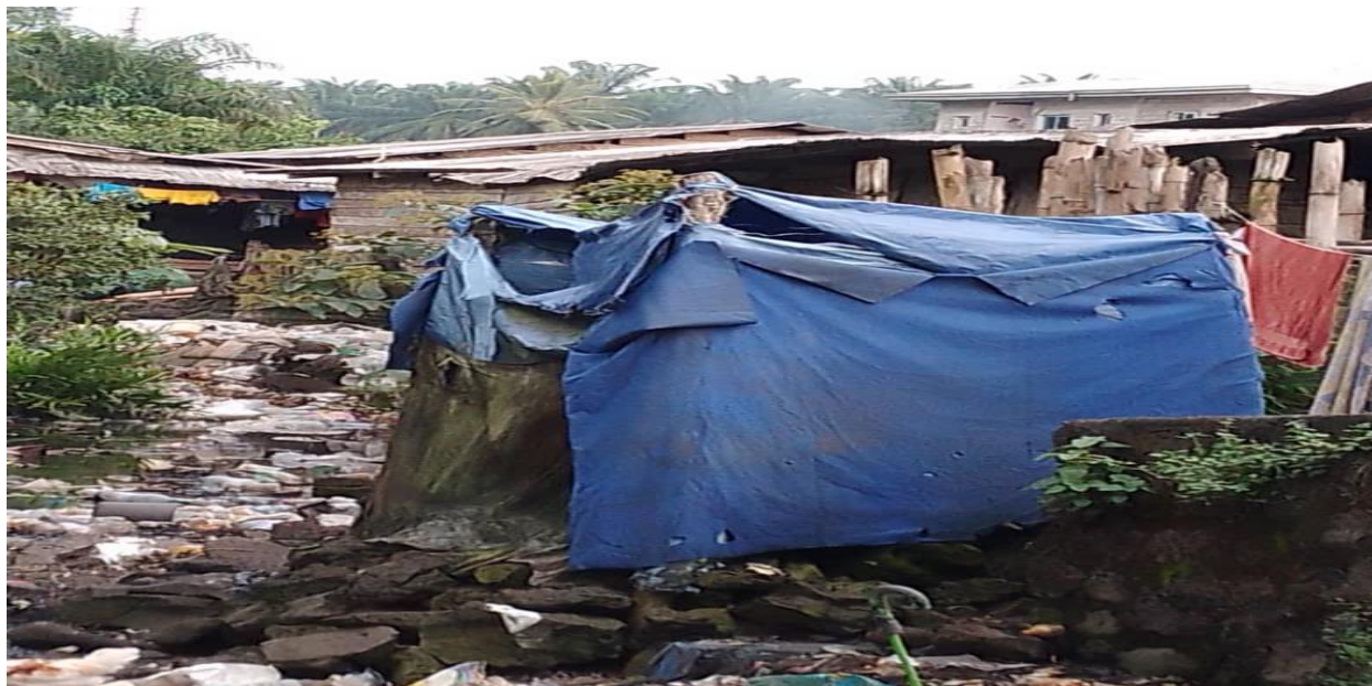
Figure 5. Bathrooms extensions constructed to enhance privacy in workers camps
