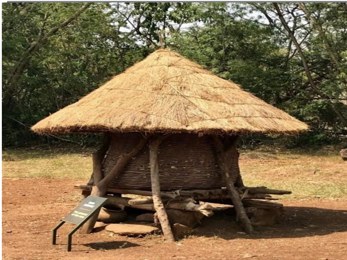
Figure 1. Traditional pole and reed granary used in eastern Zambia
