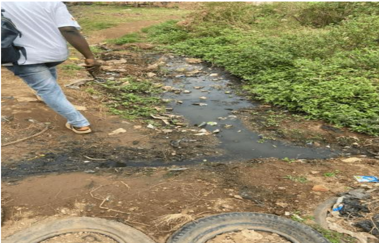
Fig. 8: Image showing dirty and stagnant water due to lack of drainage
