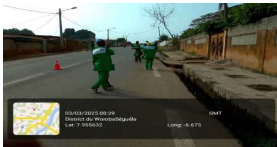
Photograph 2: Gutter cleaning agents and Cleaning in the middle of the job
