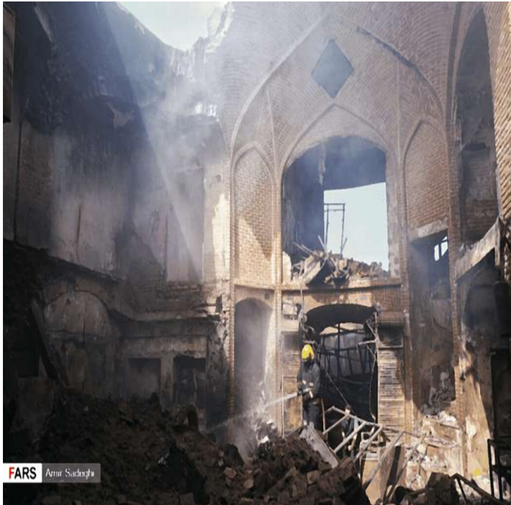
Figure 3: Fire damage at the historic Tabriz Bazaar following the fire of 8 May 2019. Photograph by Amir Sadeghi
